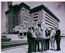
As it looked during construction
